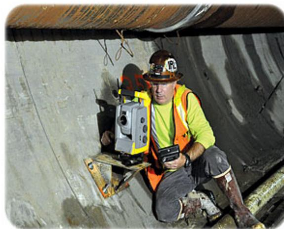
*Project Surveyor Sean Fitzpatrick, PLS, operates a Trimble S6 in the Bay Tunnel. Remote control and automated pointing enables him to quickly capture precise measurements to tunnel control points.*
