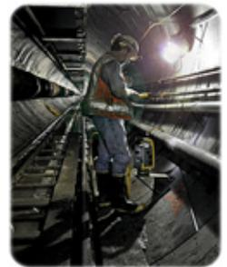
*Working deep beneath San Francisco Bay, Party Chief Russ Mello prepares to collect survey data. Precision measurements and analysis produce millimeter accuracy for guiding the tunnel boring machine.*
